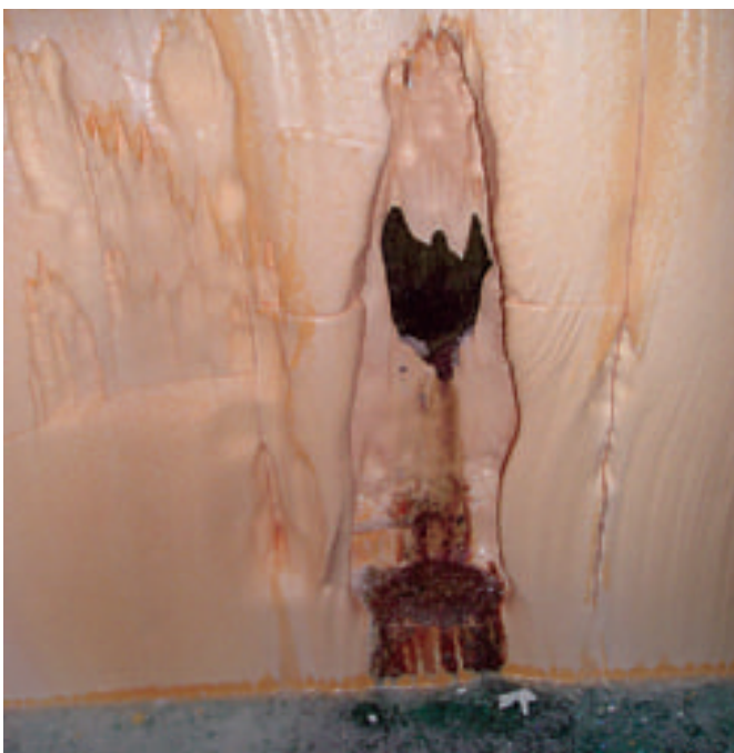
Internal wear of a melting end soldier block.
